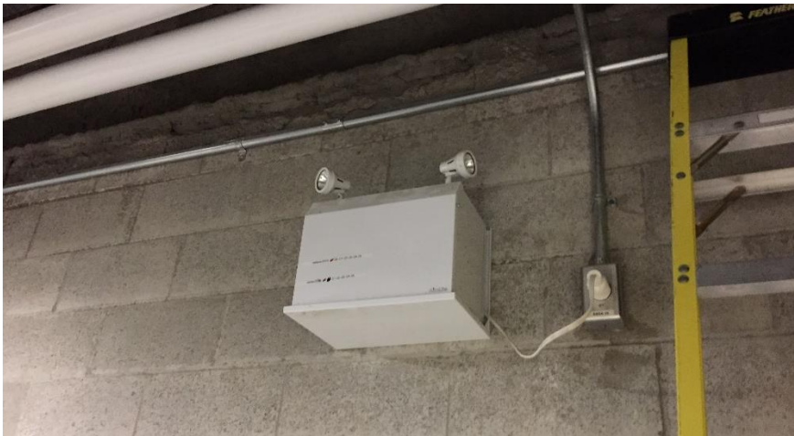
Photo 5: View of the lead-acid batteries present in Room 532C.
