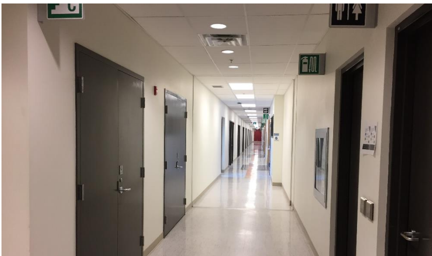
Photo 3: View of typical hallway finishes.
