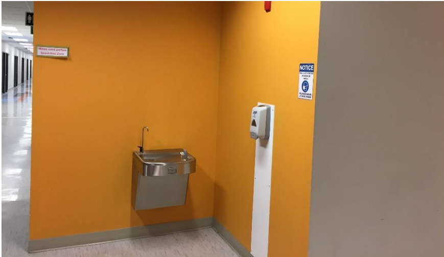
Photo 4: Typical view of ODS containing water fountain
