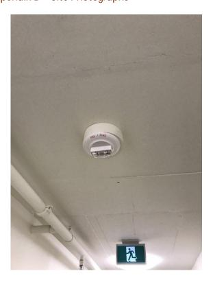
Photo 1: Reprenstative view of the smoke detectors containing small amounts of isotope Americium 241, observed throughout the subject building.
