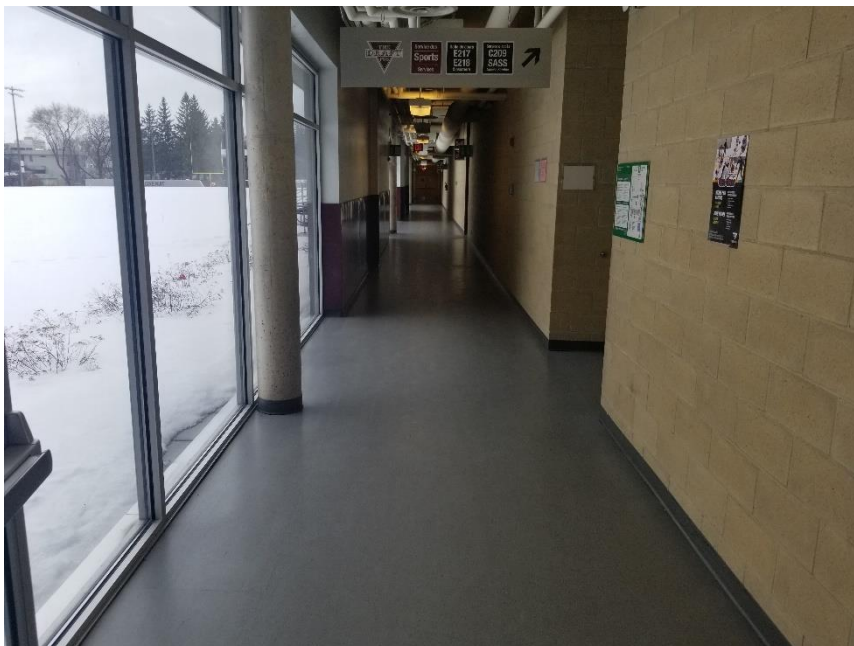
Photo 2: Typical view of finishes observed throughout the subject building.
