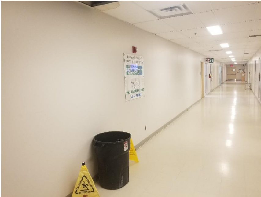
Photo 1: Typical view of finishes observed throughout the subject building.
